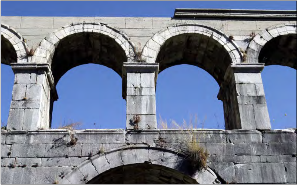
Fig. 6: Detail from the Pollio aqueduct bridge with inscription.
