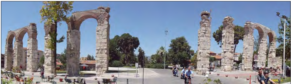
Fig. 26: Highest pillars of the Justinian Selçuk aqueduct bridge at Atatürk square. In front of the rightmost pillar is a suterasi-tower from the 14 th century.
