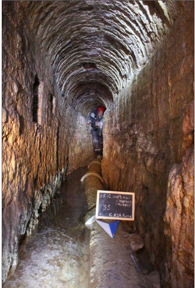
Fig. 22: Inside the Kalafat / Ayhan tunnel.
