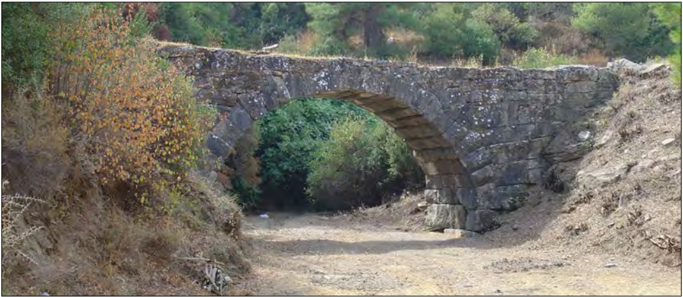
Fig. 5: Büllükdere Bridge of Aqua Throessitica.
