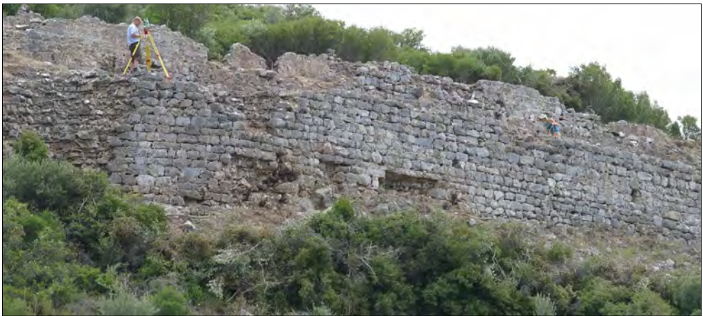
Fig. 14: Difference between Hadrian aqueduct (below) and Antonine aqueduct (above) at a highly preserved area in section XVI.
