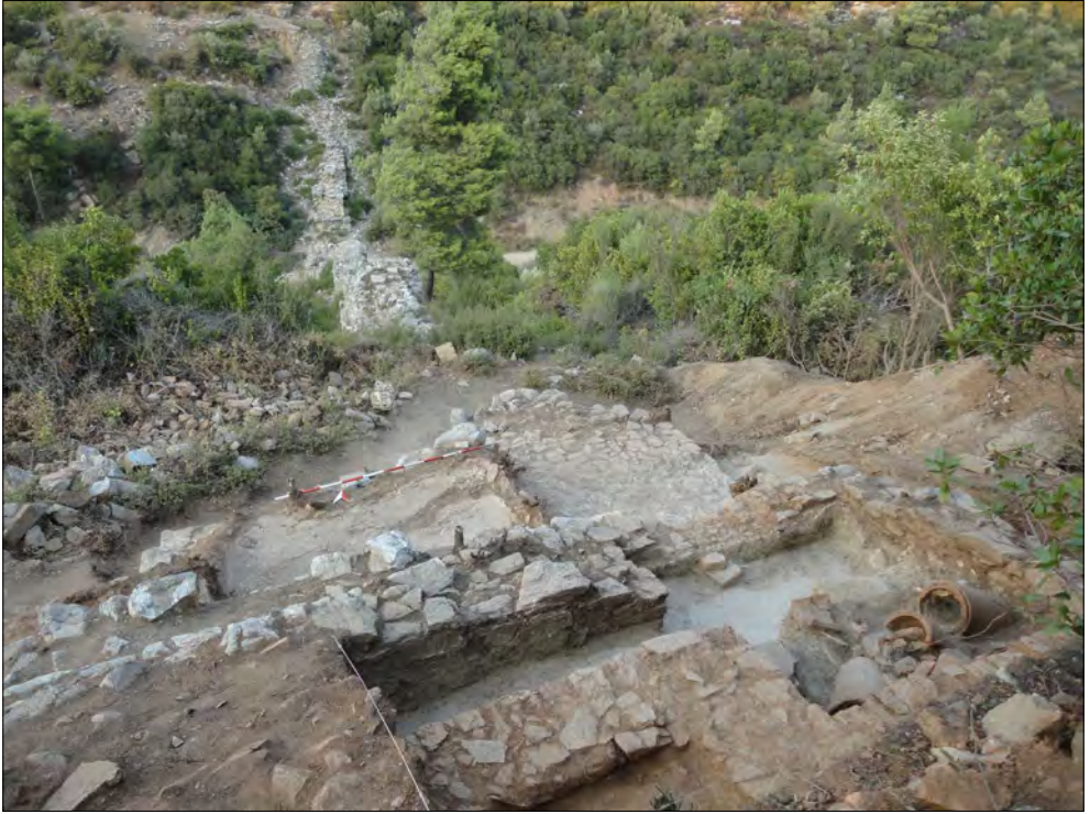
Fig. 19: Bahçecikboğaz siphon-bridge with Hadrian header tank (below) with the waste of the unneeded terracotta pipes at the place of the double basin of the Antonine header tank, the venter in the middle and the ascending ramp at the opposite valley side.
